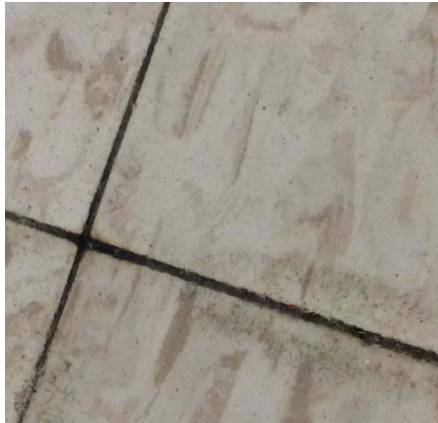
CLASSROOM FLOORING REPLACEMENT AND DEHUMIDIFICATION
