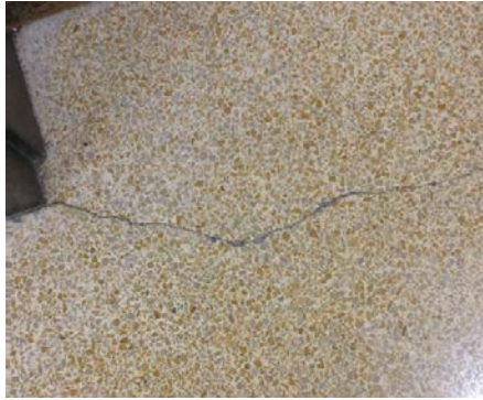
REPAIR CRACKED TERRAZO
