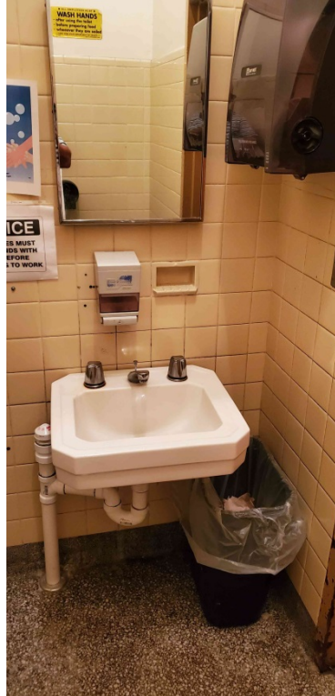
Custodial Toilet Room
