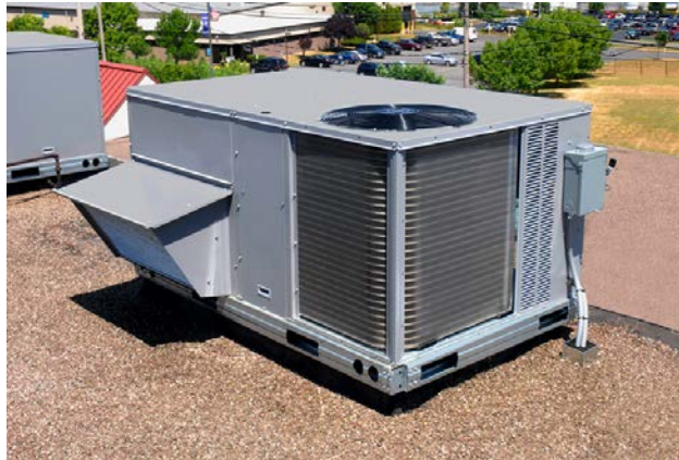
ADD AIR CONDITIONING TO 10 2 ND FLOOR CLASSROOMS
