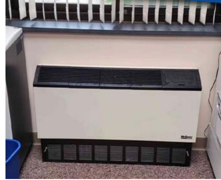
DISTRICT OFFICE HVAC REPLACEMENT
